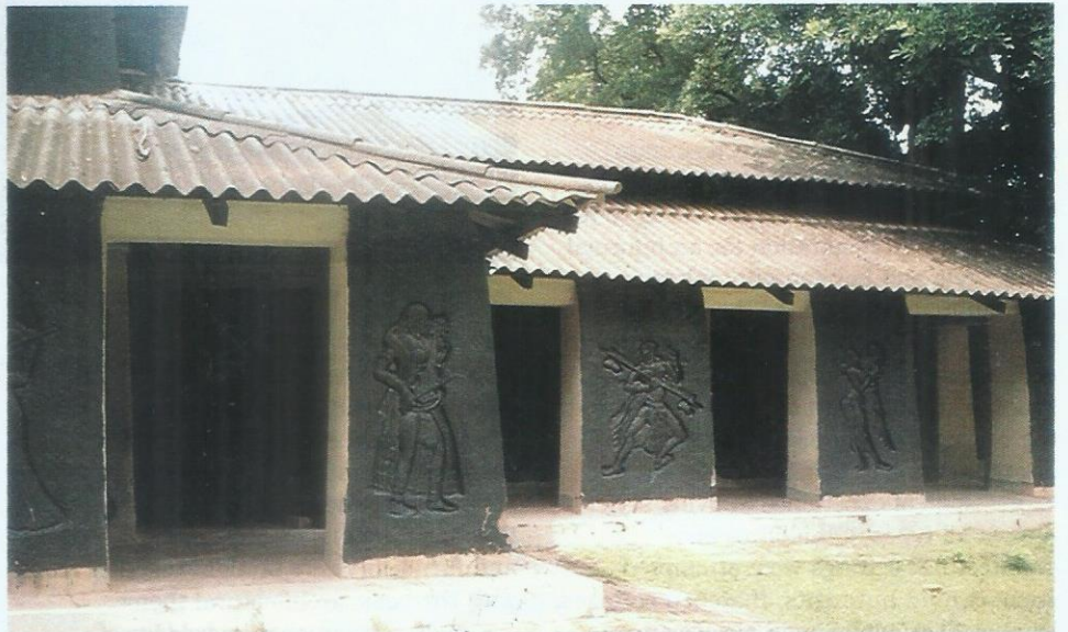
Top Udayan — art-architecture ethos Above Kala Bhavan hostel (mud architecture)
